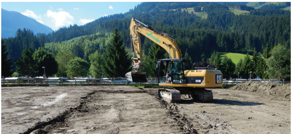
Figure 29: A positive example of soil treatment: The loosening of compacted soil followed by filling of underground and top soil in layers (Photo: Thomas Peham).
